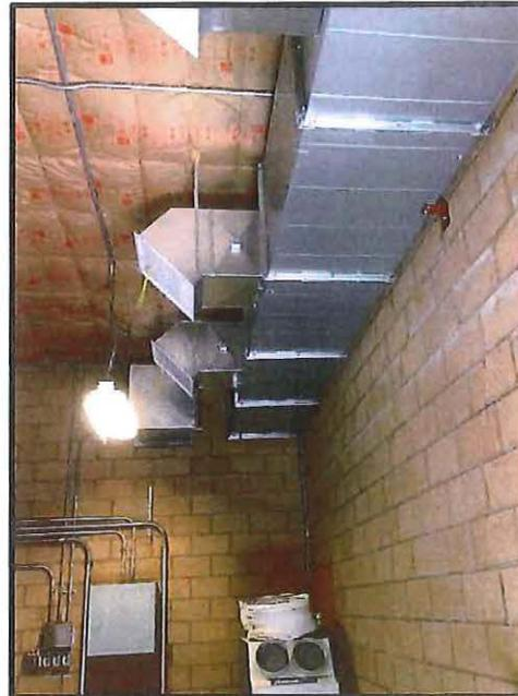
Installed ceiling insulation and AC air ducting
